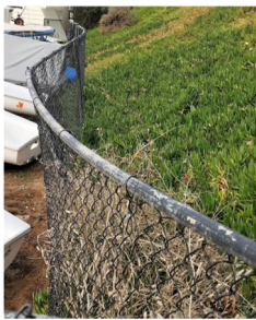
Damaged boat yard fence
