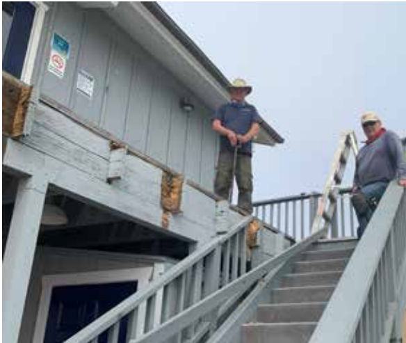
Our awesome deck volunteers John Burgener and Mark Hilden during deck demolition, notice the extensive rot in the exposed joist ends.
